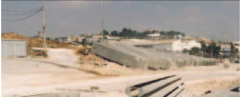
Lying sections of the wall
